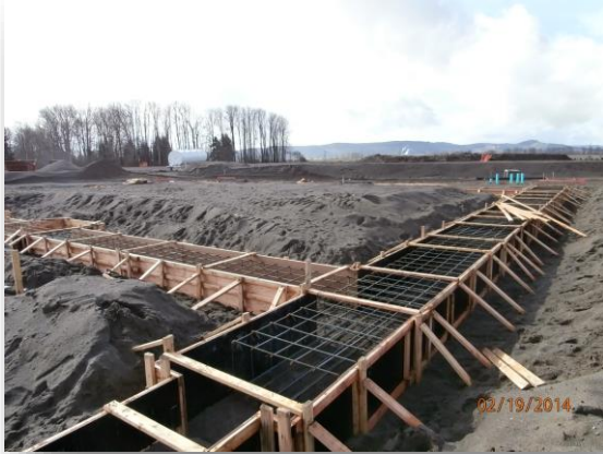
Form work at north edge of aux. Gym
