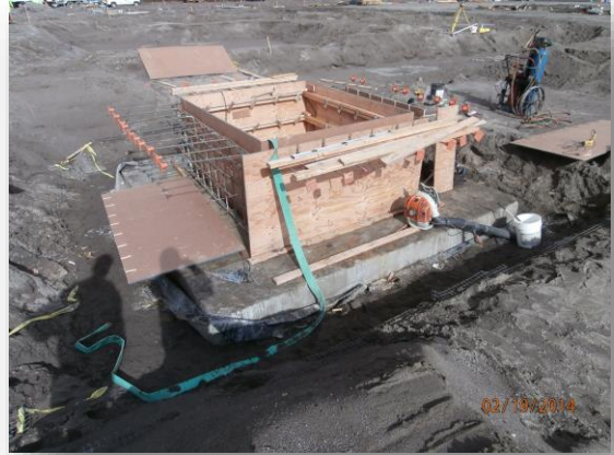
Form work and footings at elevator pit
