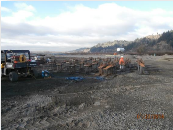
Steel embed plates at footings for structural super structure
