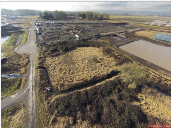
Aerial photo – looking south from NE corner
