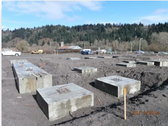
Footings at North Classroom Wing
