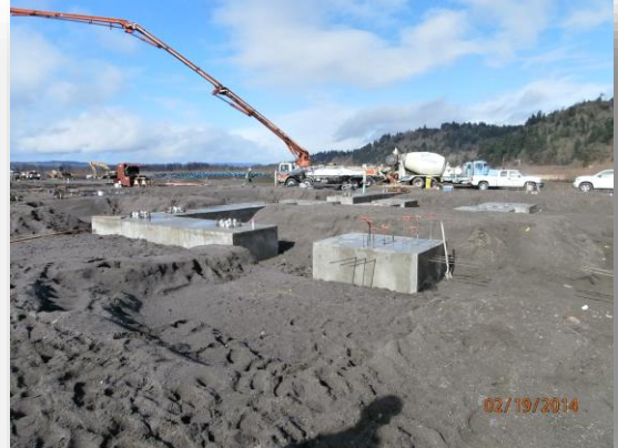
Footings at North Classroom Wing
